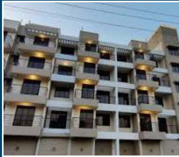
Konark Relators & Builders
