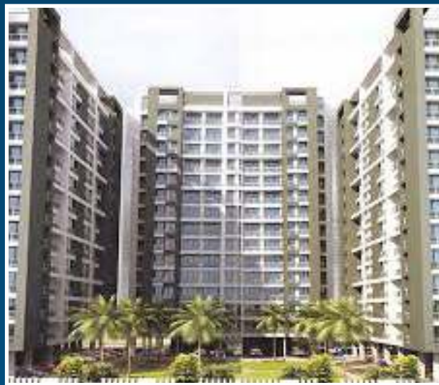
Puraniks Builders & Devlopers
